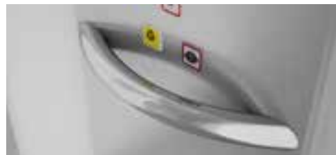
Curved handrail over COP
